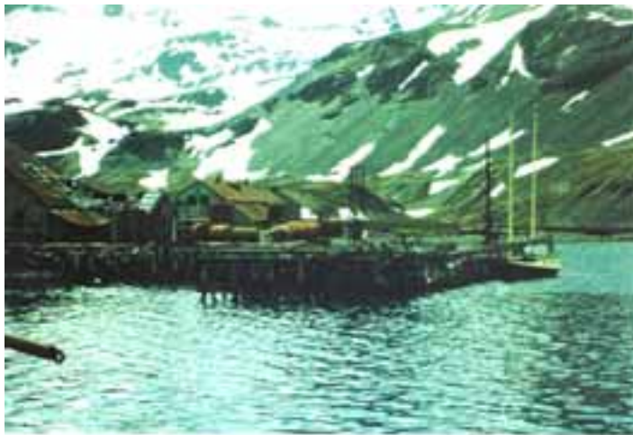
STORMNESS HARBOUR, THE MAIN DOCK - LOOKING N
