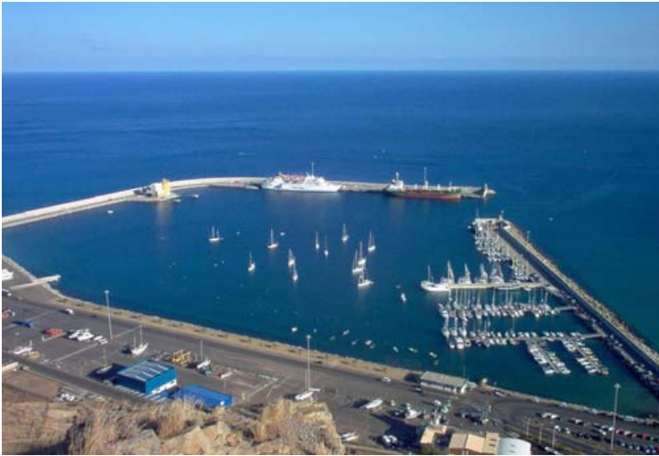
The harbour at Baía de Porto Santo, showing the additional marina pontoons
