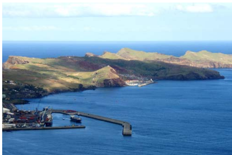
The new breakwater at Caniçal seen from the northwest, with Quinta do Lorde Marina behind
