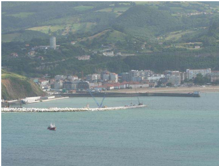
New large harbour under construction Peter Adam – Summer 2008
